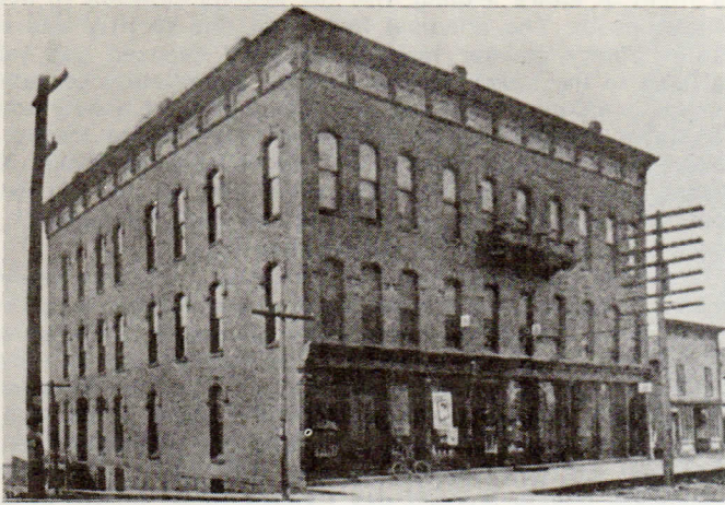
An unlovely view of the Grandin's domain circa 1904. It is tempting to believe that the poster seen in the drug store window advertised an attraction at the opera house.
